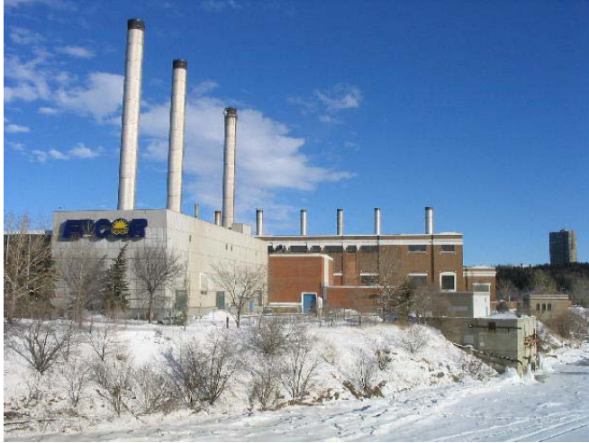
Figure 2: The EPCOR power plant in Rossdale
